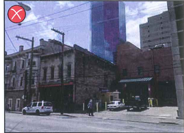
Utilities not hidden become unsightly to both pedestrians and motorists passing by.
