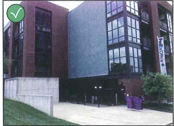
Utilities can be hidden even without completely blocking them out of sight by simply blending them into their context.
