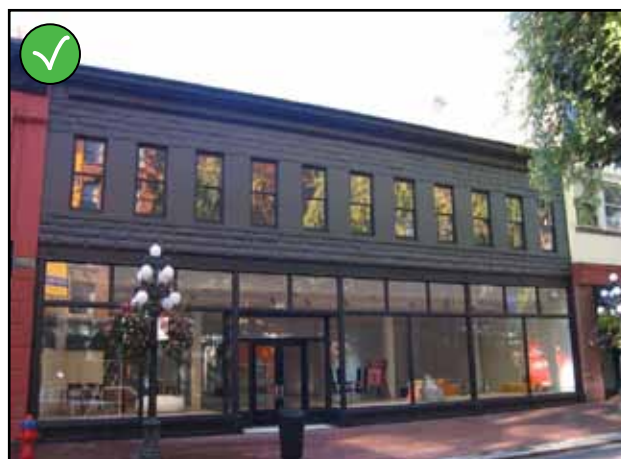
Creating properly scaled storefronts enhance the building and the pedestrian experience.
