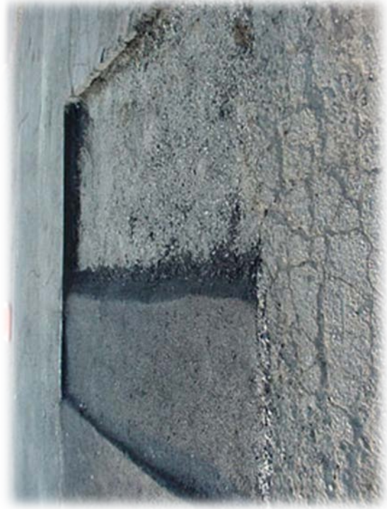
Asphalt Patching
