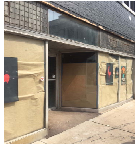
Exhibit C- Existing Recessed Entry
