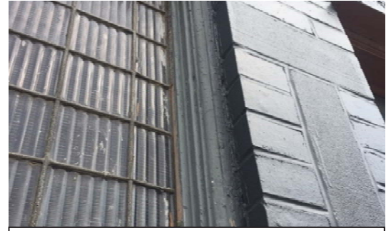
Exhibit G- Existing Brick Molding
