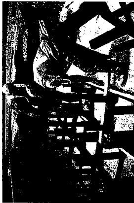
Construction photo showing placement of subsurface integrated tree and stormwater system (Silva Cell by Deeproot).
