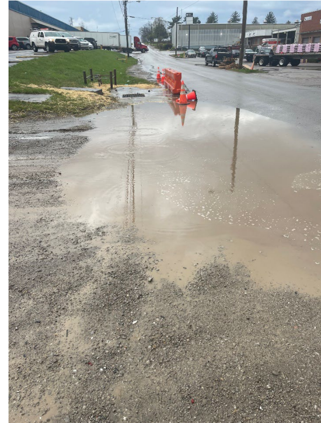
Lisle Industrial Road
