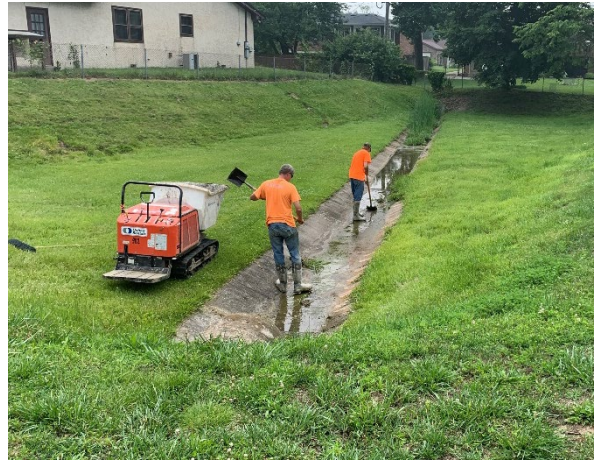
Cleaning Concrete Flumes
