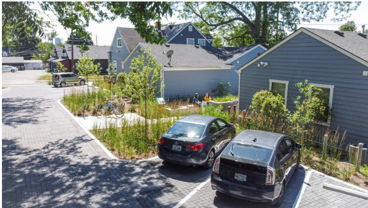
FY20 900 Block of North Limestone Stormwater Retrofit – Pervious Pavement, Rain Gardens, Bioswale, Water Walk Complete (ASLA Award of Excellence)
