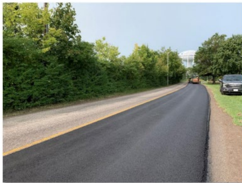
Figure 1 – REARM constructed pavement on Mercer Rd looking west
