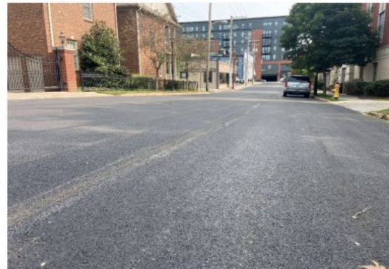
Figure 3 – REARM constructed pavement on Cedar St looking southeast towards S Upper St
