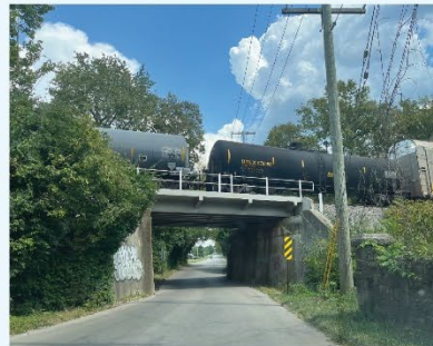
Sandersville Road under Rail Crossing
