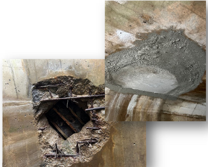
Repaired a Hole In Town Branch Culvert
