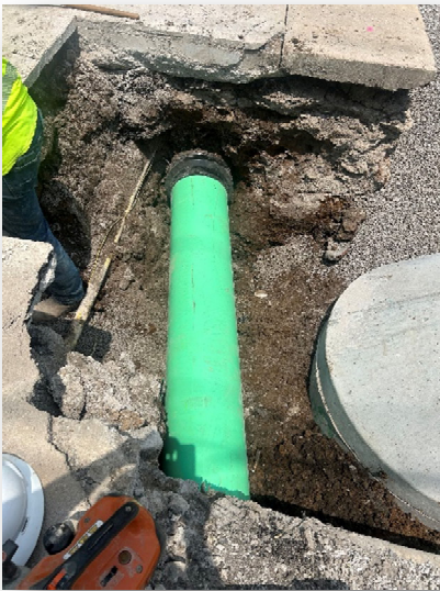
Performing a Point Repair to Fix Broken Pipe
