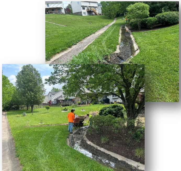
Cleaning Concrete Stormwater Flumes
