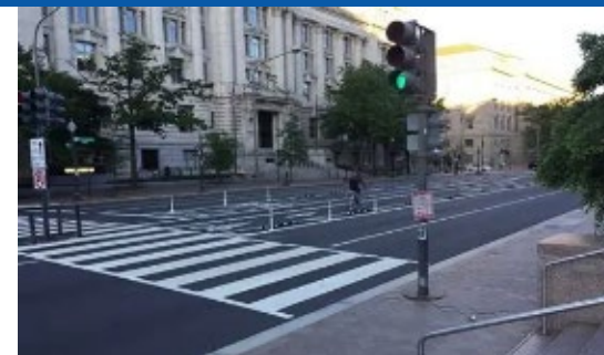
Signalized Crosswalk Study
