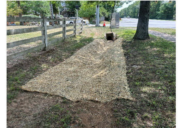
Wyndham Hills & Clays Mills (Buried Inlet – Impacted Storm Pipe)
