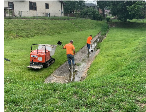
Cleaning Concrete Flumes
